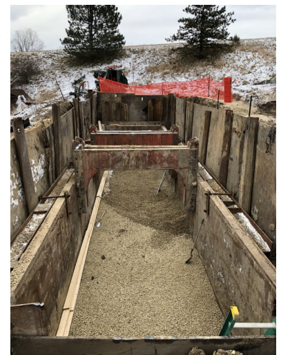
Bore pit under I69
