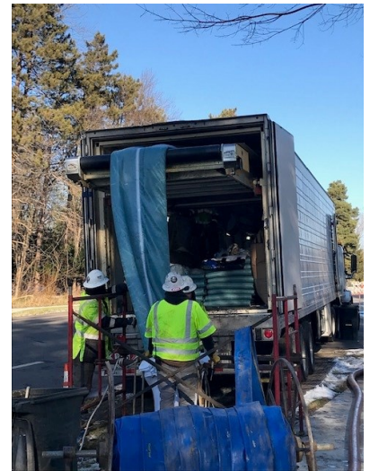
Insituform Liner installation
