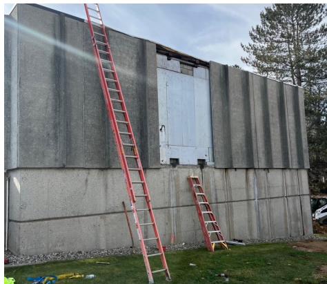
TE wall removal
